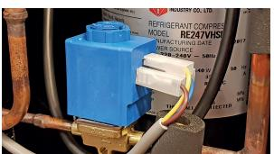
**6.** Ensure that the capillary tubes of the thermo valve are secured with insulation and strips as shown.
